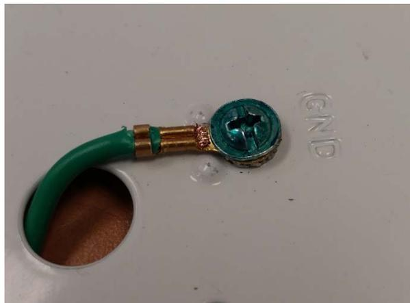
Figure C: Grounding Assembly
